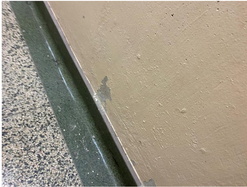
Photograph 1: View of cream paint containing high concentration of lead within Corridor (53631).
