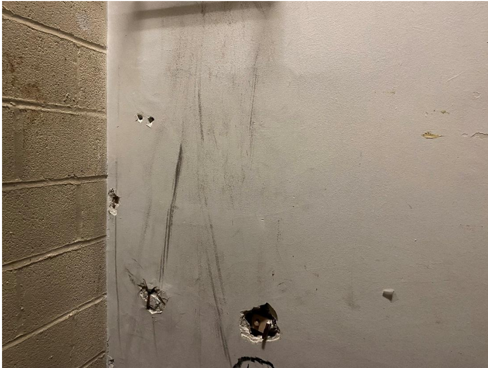
Photograph 3: View of off-white paint containing high concentration of lead within Stage (5513).
